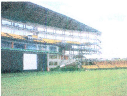
Figure3.3 : the linear form of the grand stand meeting the curved and irregular form of the lower stands
