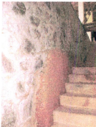
Figure3. :textures of the tunnel
