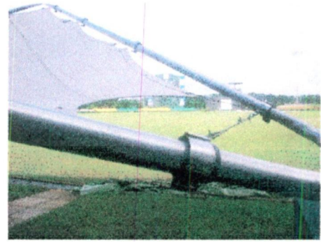
Figure3. : detailing of the fabric roof, sleek and slender
