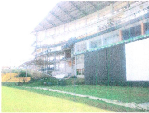
Figure3. : the scale and proportions of the lower stands with tensile roof is much smaller than the grand stand scale and it is the human scale. But the detailing was able to bring this scale of the grand stand back to human scale
