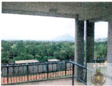
Figure3. : upper floor balconies provides view of the
