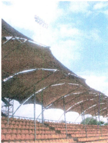
Figure3. : the tensile roof reminding the temporary structures
