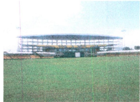
Figure3. : the colours of the natural setting is added to the built form by almost invisible grand stand.
