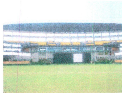
Figure3.2 : the curved form of the grand stand emphasising horizontality in this elevation.
