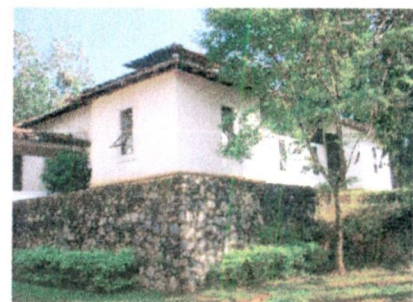
Figure3. :rubble wall exposed to makes the building part of the place
