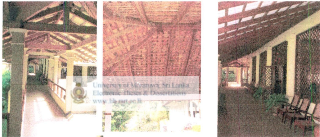
Figure3. :roof is detailed using exposed timber to evoke similar feelings under the trees
