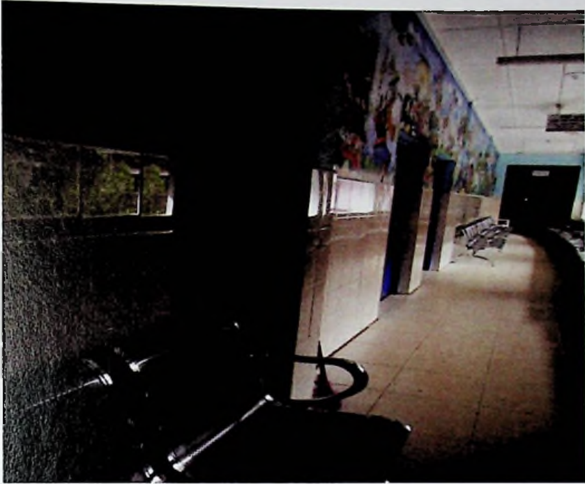
Figure 3.18: A Lobby area finished with locally manufactured tiles in OPD building at LRH renovated with local funds
