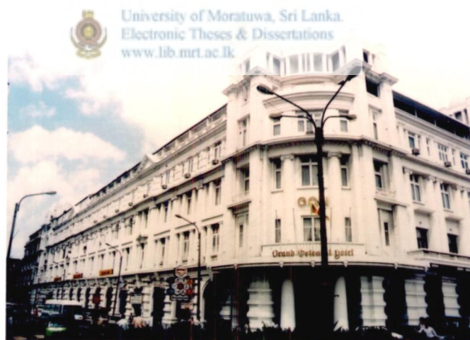
Fig.82 The Colonial Building Facades of the West Elevation.
