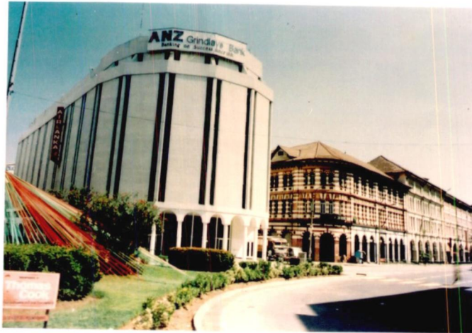
Fig.83 Stands with the Monotonous Building Façade
