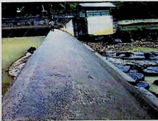
Figure 9: Weir & Intake Structure of the Way Ganga MHP
