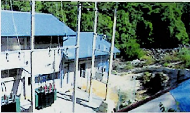
Figure 12: Power House of the Way Ganga MHP
