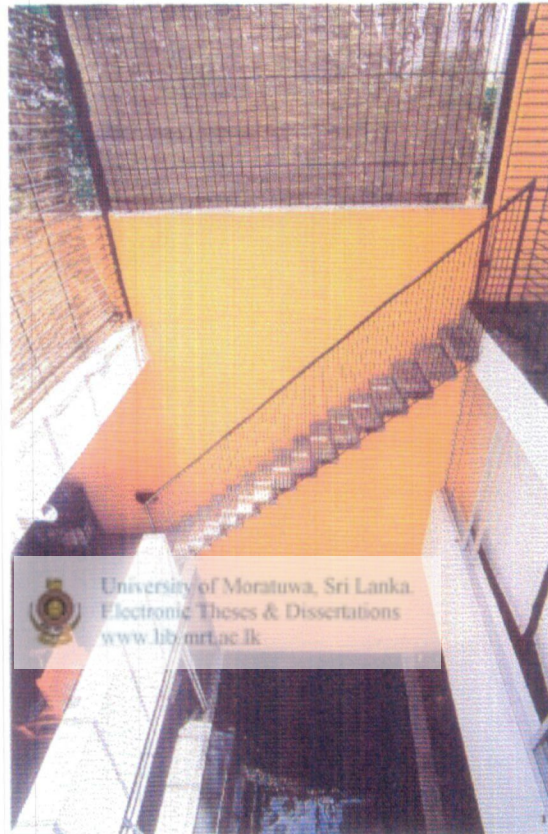
[Fig.101] Open rise steel and timber staircase
