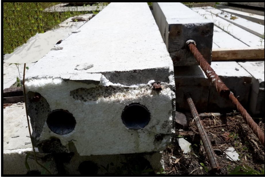
Figure 2-1: 150×250mm column with the provision of two 40mm grout holes (left) and three 150×150mm columns with T25 anchor bar fixed (right)
