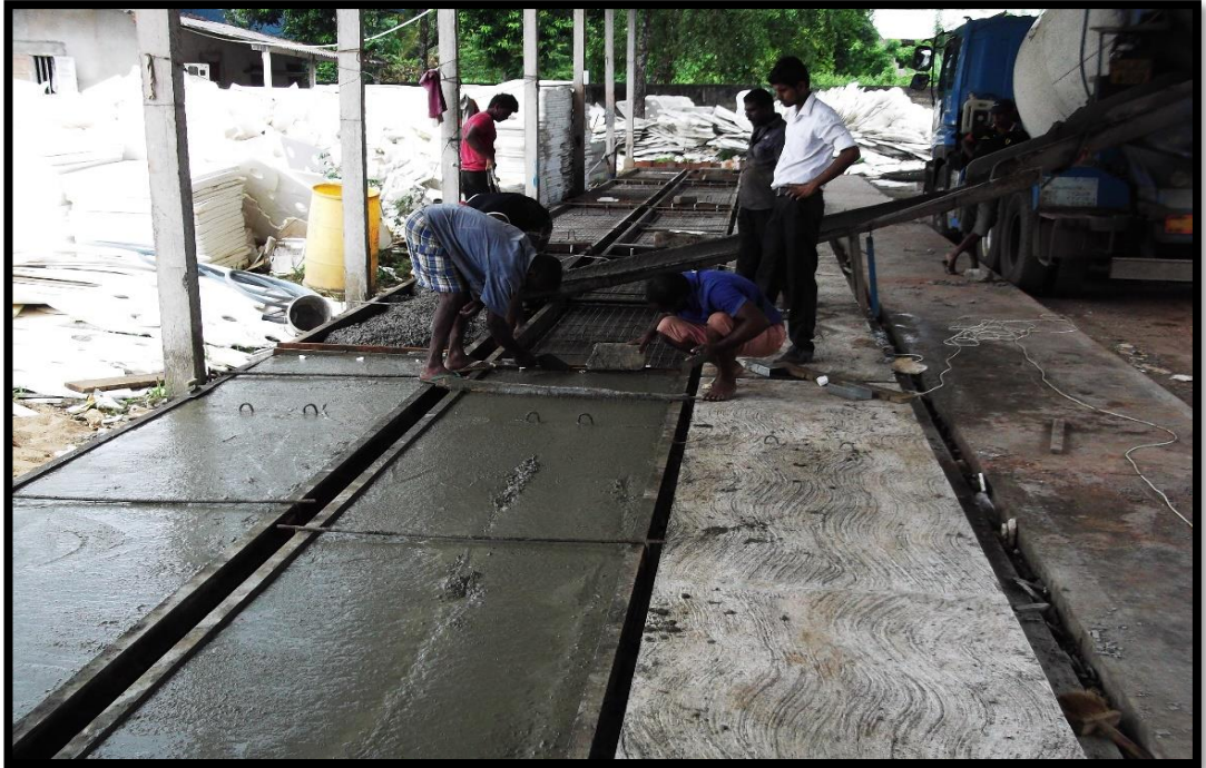
Figure 2-4: Concreting of slab panels with at the casting yard at Ekala (2015)
