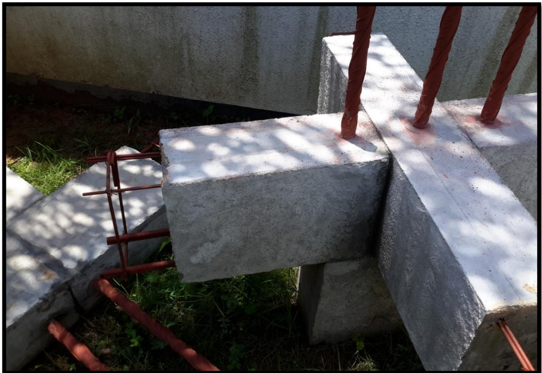
Figure 2-8: A typical beam-column connection (Fernando,2016)
