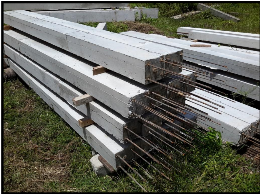
Figure 2-2: 150×150mm columns- stacked at the yard with untrimmed prepressing strands
