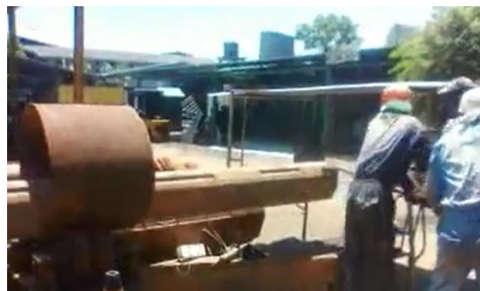
Figure 57: Manual Rotation of Kelly bar by workers
