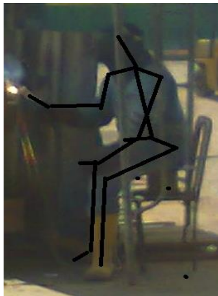
Figure 59: Worker performing repair
