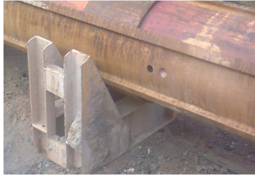
Figure 7: Fix stationery mounting in workshop CML-MTD Construction Ltd.
