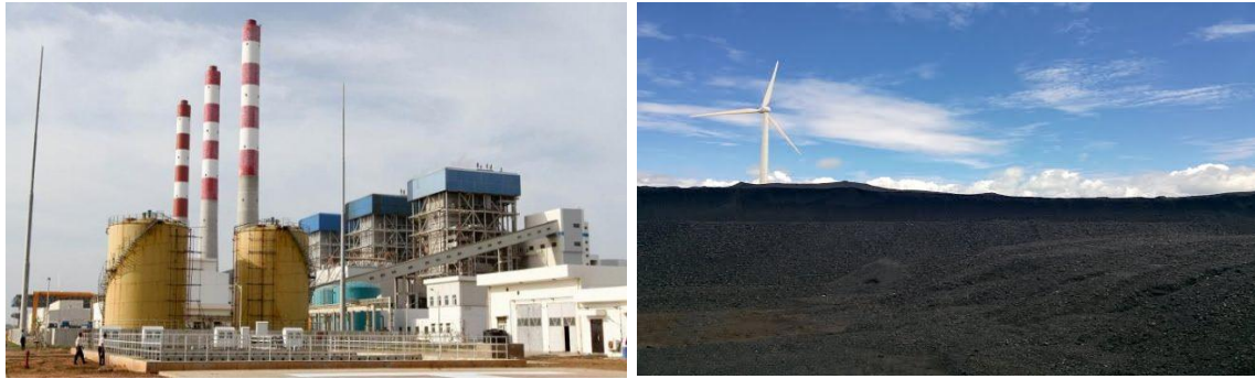
Figure 1.1: Coal Power Plant & Ash Mountains in Sri Lanka (Lakvijaya Power Station)
