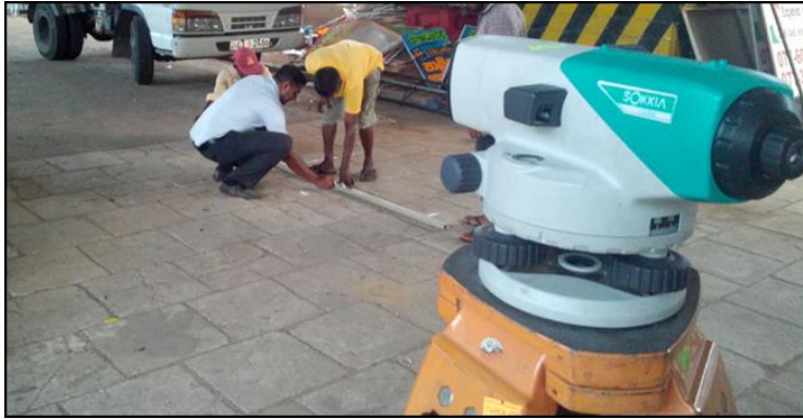
3-2 Marking guidelines and preparing ground surface
