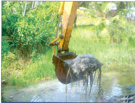
Tsunami Debris were Removed Using Machines
