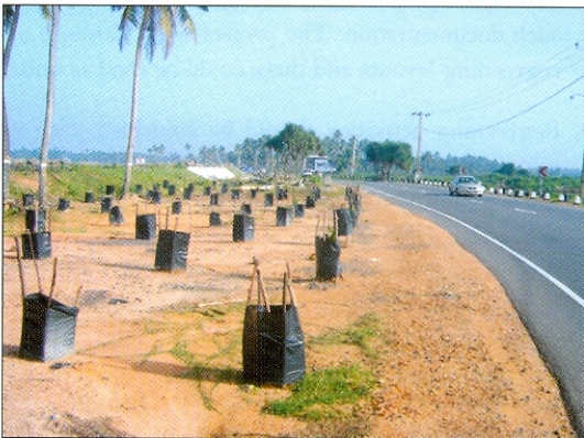
Polythene Covers were used for Plant Protection
