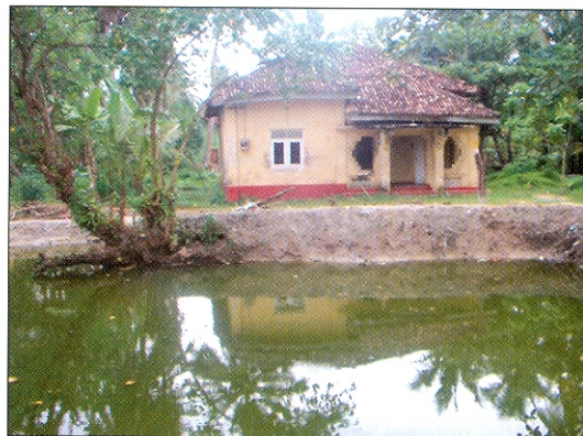
Earth Bunds were Formed Around Rehabilitated Coral Mines
