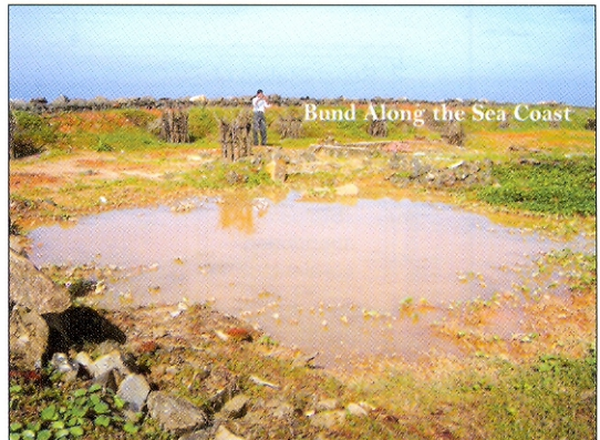
Bund Along the Sea Coast Obstructs Natural Drainage
