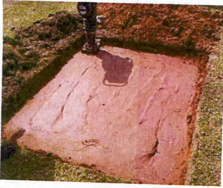
Figure 6.4 Compacted ant clay layer and holes driven in
