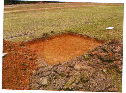
Figure 6.6 Excavated pit for the pitch model
