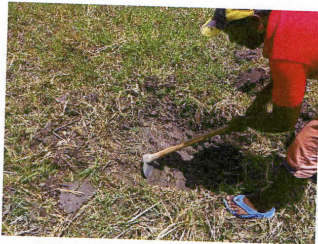
Figure 3.2 Excavation of pits in clay deposits
