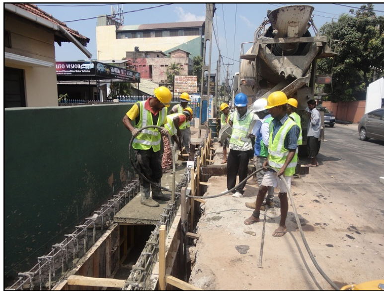
Figure 3-14: Existing drain walls raising to provide foot-walks
