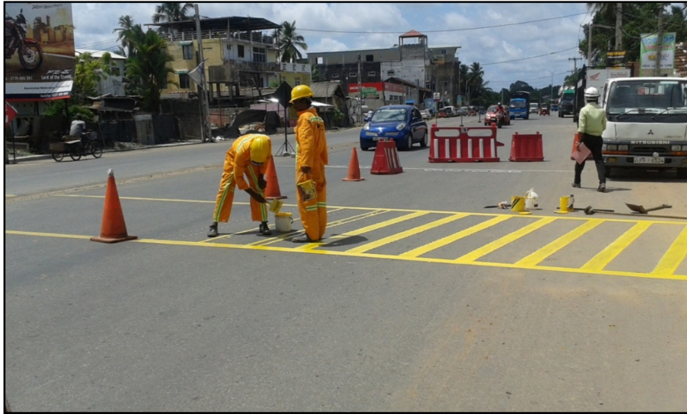
Figure 4-6: Temporary Pedestrian Crossings at B084 Road Project
