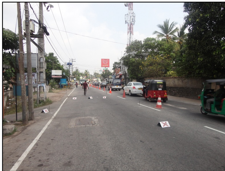
Figure 3-15: Single pile traffic allowed in construction zones
