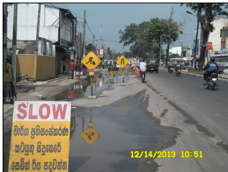
Figure 3-5: Properly arranged temporary sign boards
