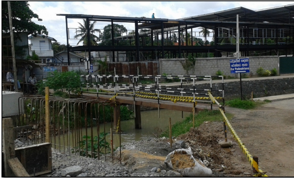
Figure 4-5: Temporary pedestrian Bridge at B084 Road Project
