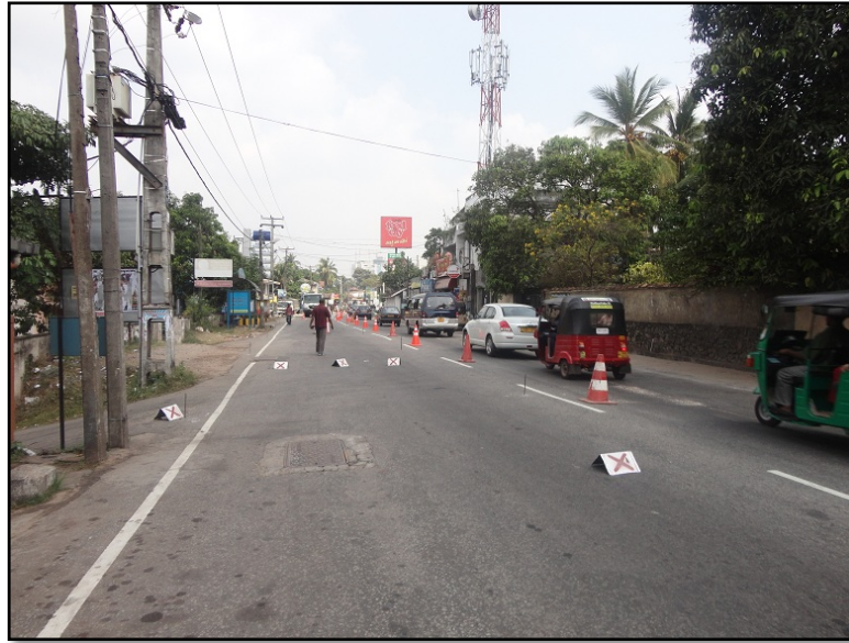
Figure 4-16: Traffic Management during asphalt paving at B120 road
