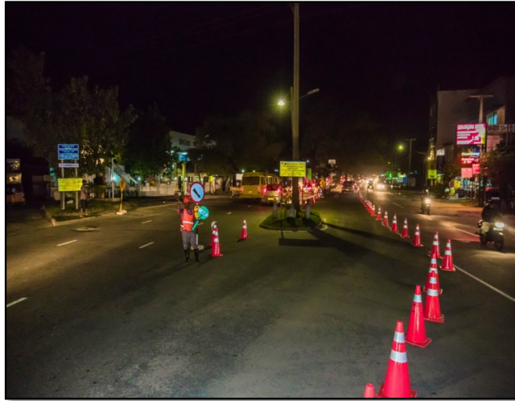
Figure 3-6: Traffic diversion during night time
