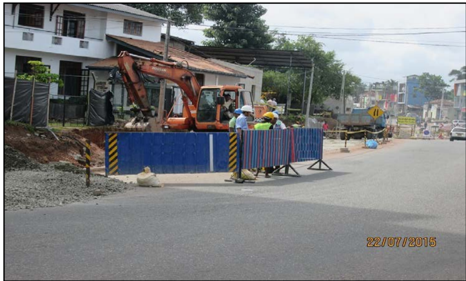
Figure 4-11: Traffic Management during culvert construction at B084 road
