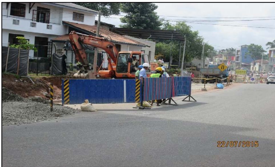
Figure 3-9: Demarcation of work-zone
