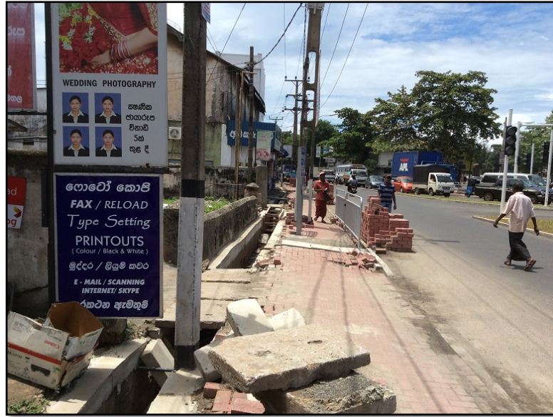
Figure 3-2: Disturbances to the Pedestrian Foot-walks
