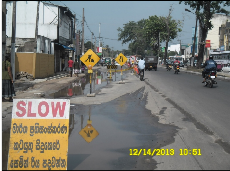
Figure 4-10: Traffic Management during culvert construction at A002 road
