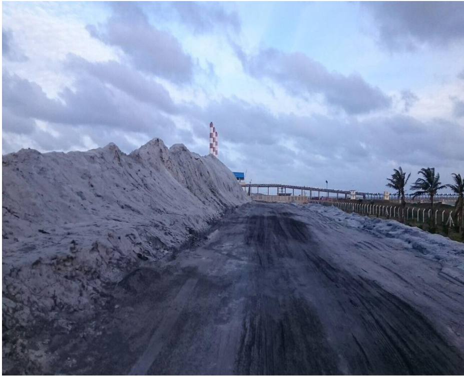
Figure 1.4: Dumped ash inside the power plant premises by wet unloading
