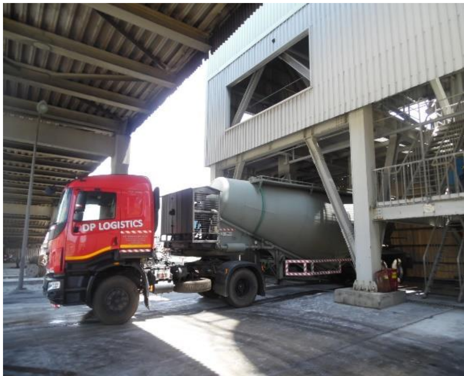
Figure 1.5: Dry unloading of fly ash for cement production
