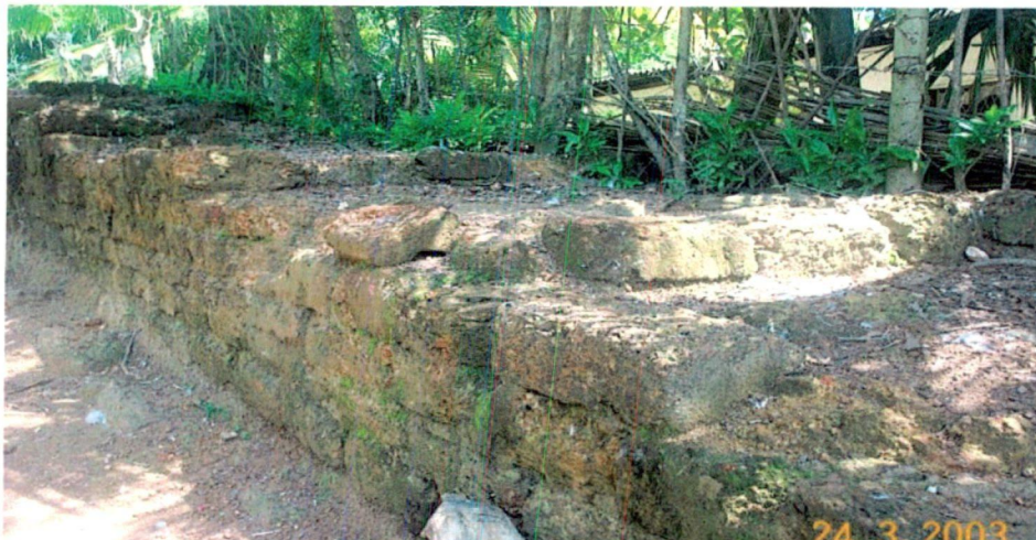
Figure 2.04 Existing situation of Rampart
