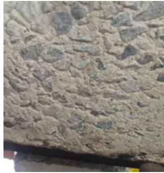
Figure 3.8: Concrete surface after surface preparation
