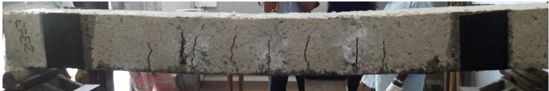
Figure 4.27: CFE2 Beam after loading
