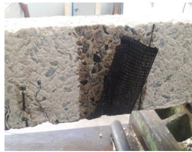
Figure 4.14: Delamination of U wrap end anchors
