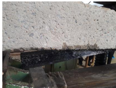
Figure 4.21: Delamination of end CFRP
