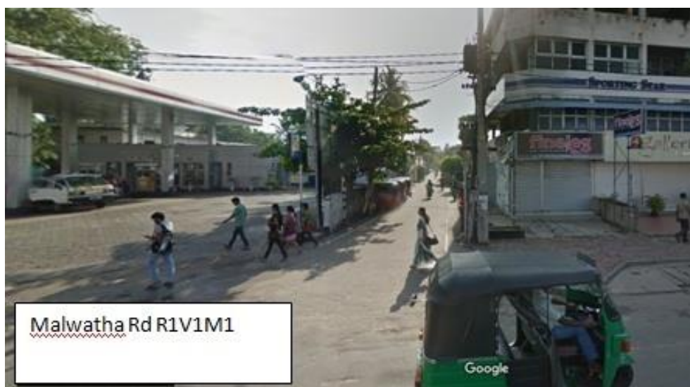
Figure 5.11: T Intersection at Malwatha Road [R1V1M1]
