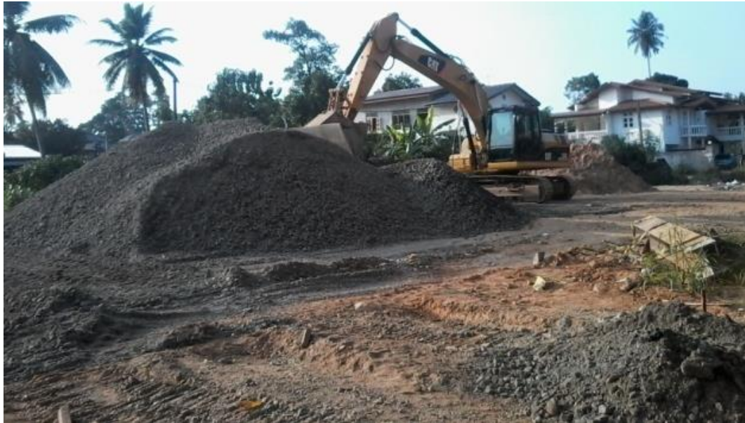
Figure 3-3 Control the MC of DGAB at stock pile
