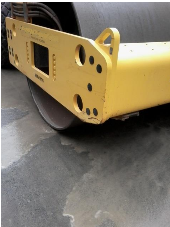
Figure 3-1 Compaction of DGAB under high Moisture Condition
