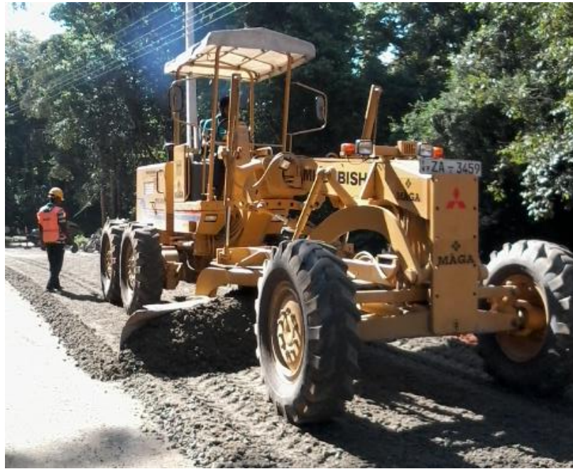
Figure 5-5 Laying of DGAB using a Mortar Grader
