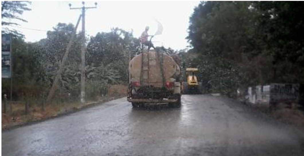
Figure 3-6 Watering on DGAB surface while compacting
