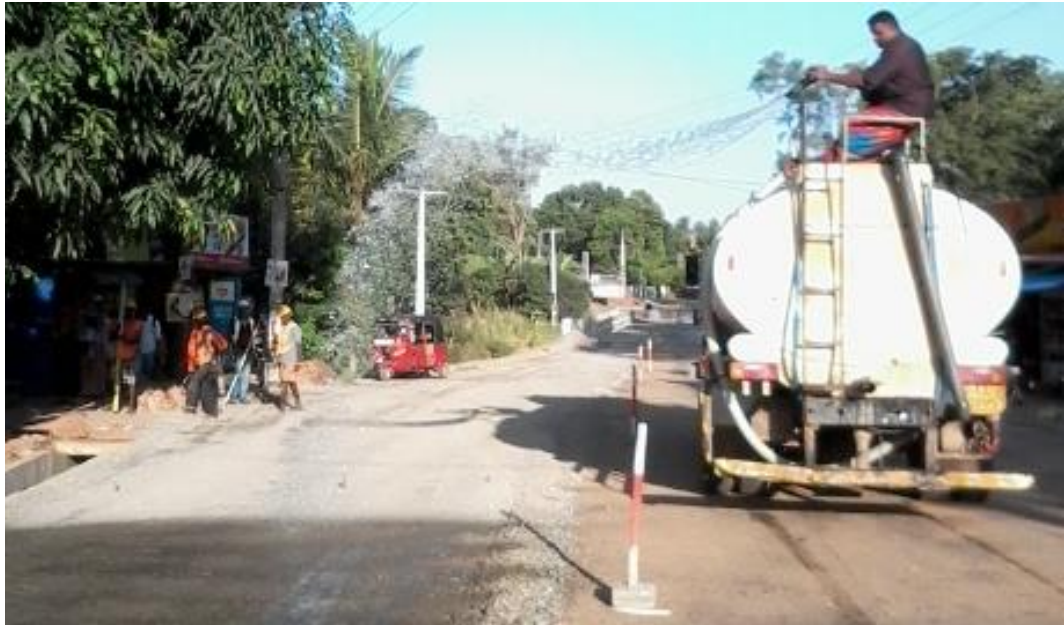
Figure 3-5 Adding water on DGAB & compacting without mixing
