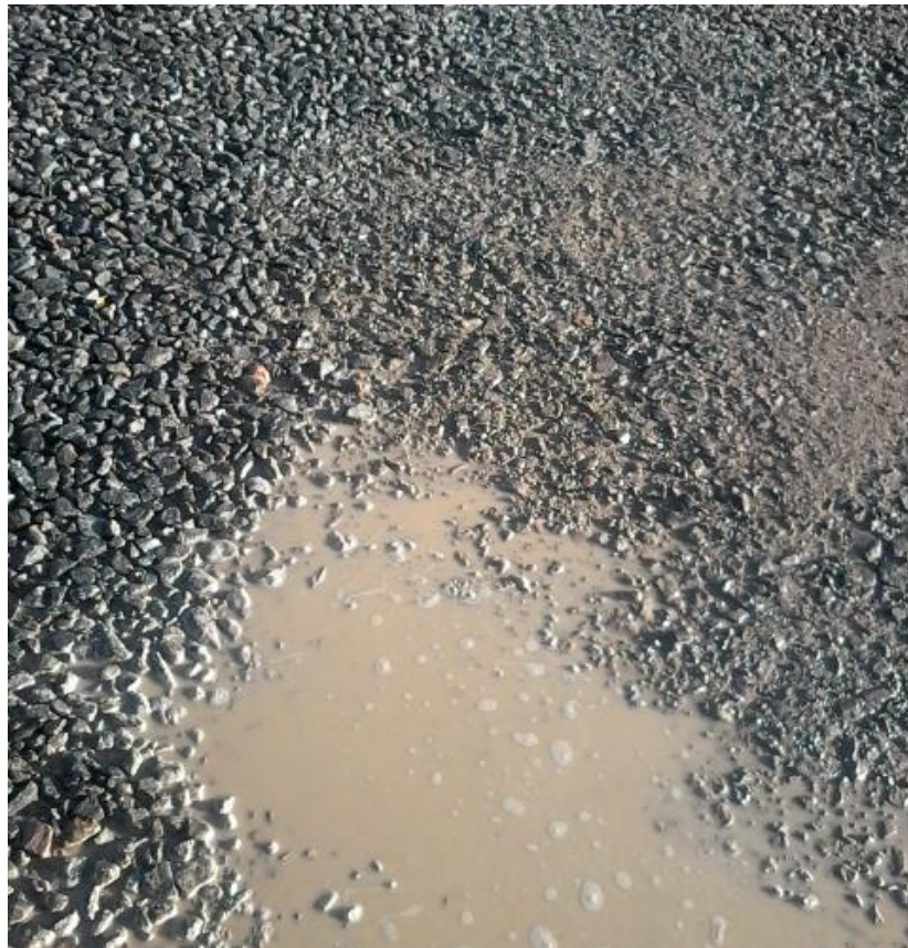
Figure 6-1 Segregation of DGAB Layer during the Compaction
