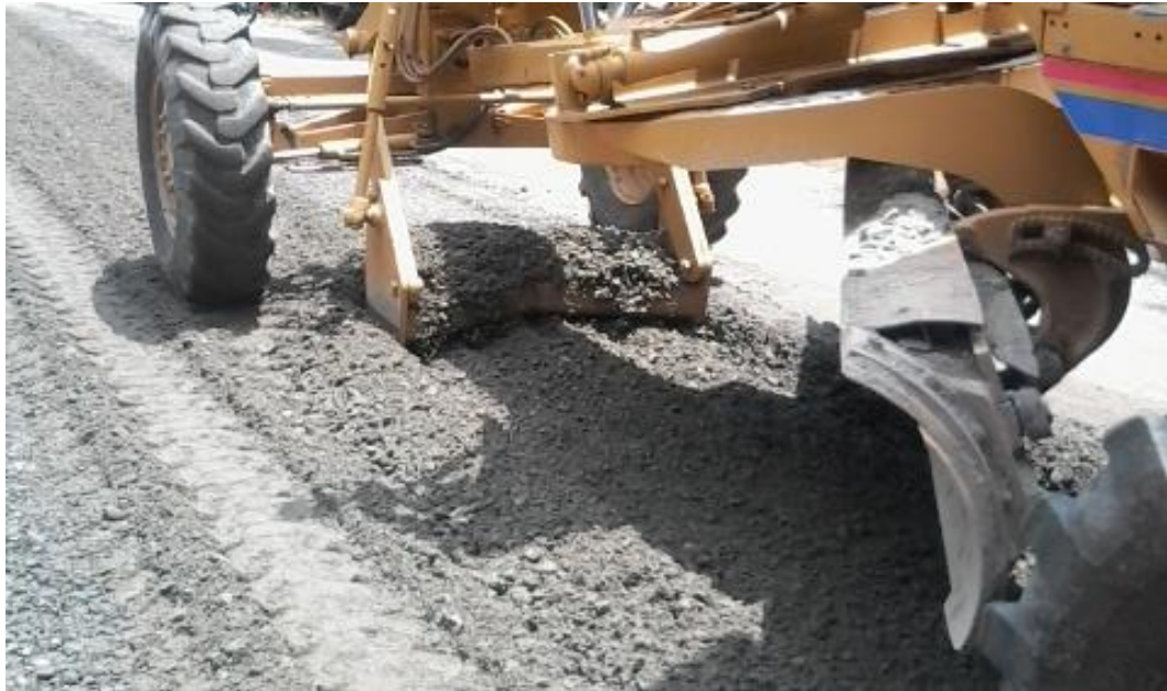
Figure 3-4 Control the MC of DGAB at Site by Mixing
