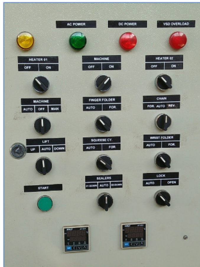
Figure 5.1: Control panel of the machine
