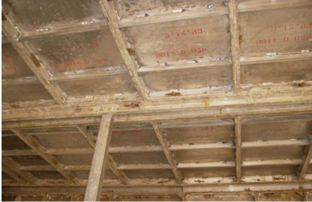
Figure 5.3: Deck Component (Patil and Prof. Desai (n.d.))
