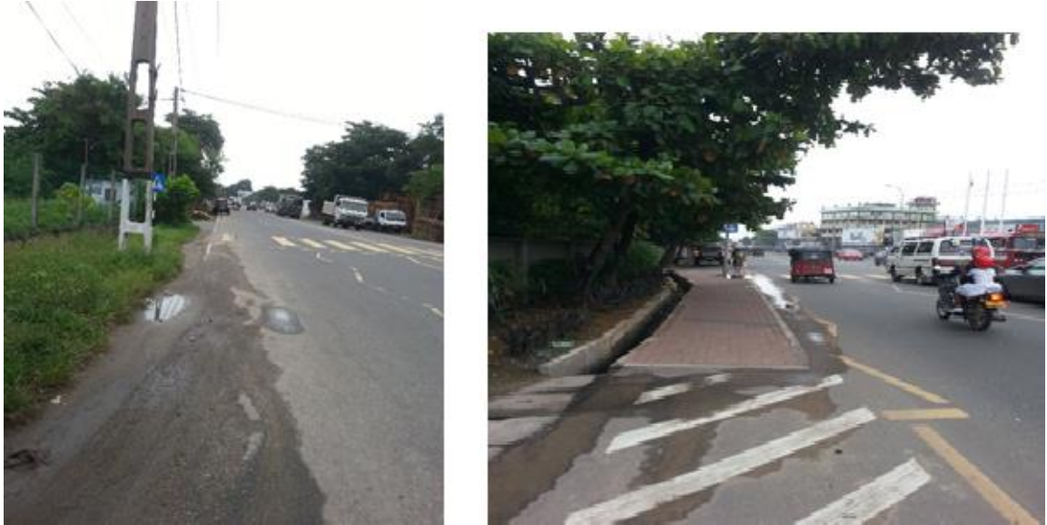
Figure 4.3: Obstruction of signboard by electric post and tree (A3 Road)
