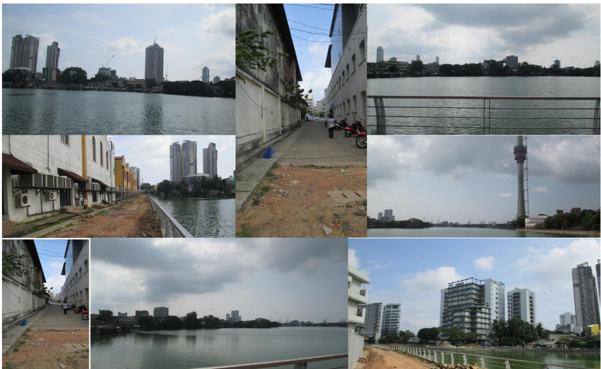
Figure 5.33: Buildings projecting out wards form Vauxhall street. , Source: Author
