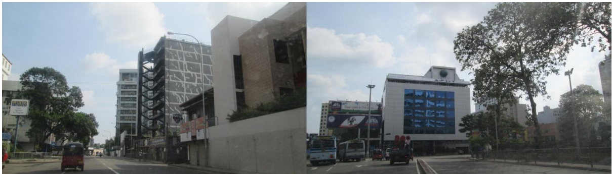
Figure 5.38: Junction of Union place. , Source: Author
