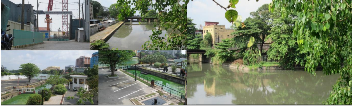
Figure 5.24: The Mc Cullum gates connecting the water body to the Indian Ocean, Source: Author
