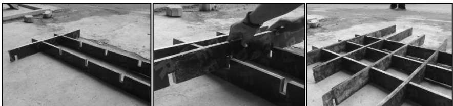
Figure 6: Form work made by plywood
