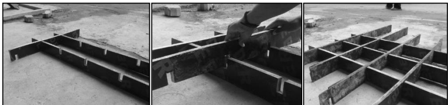
Figure 6: Form work made by plywood
