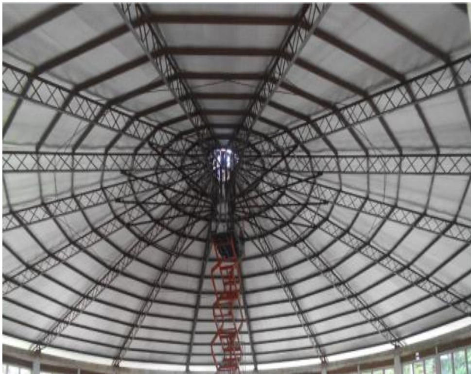
Figure 36: Roof of Kulasinghe auditorium
