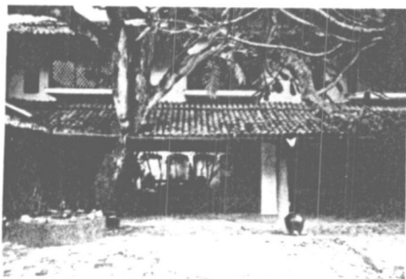
Fig 82 A house with large tree, Ena de silva house, Colombo.
