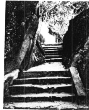
Fig 60 A pathway with steps Ritigala Monastery complex
