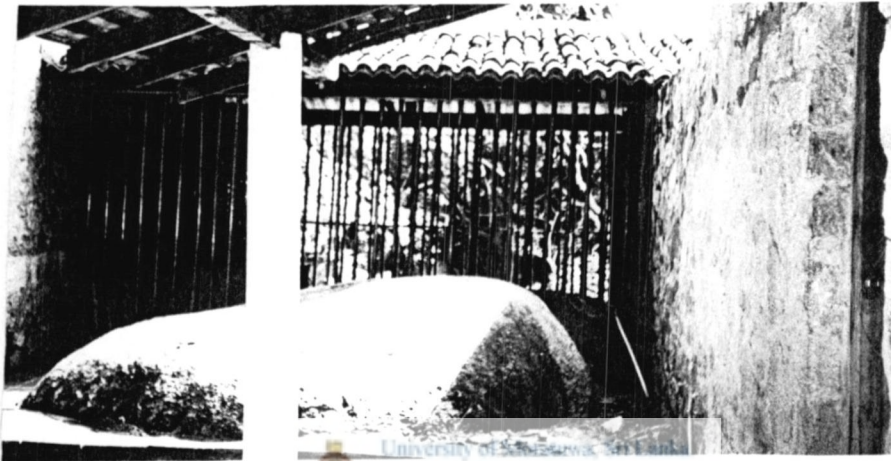
Fig 95 Isolated boulders create a entrance lobby for the bed room wing
