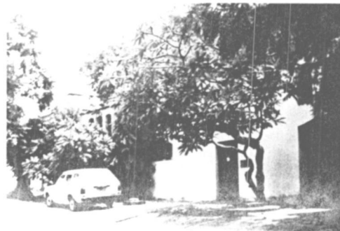
Fig 83 Ahouse at fifth lane Colombo.
