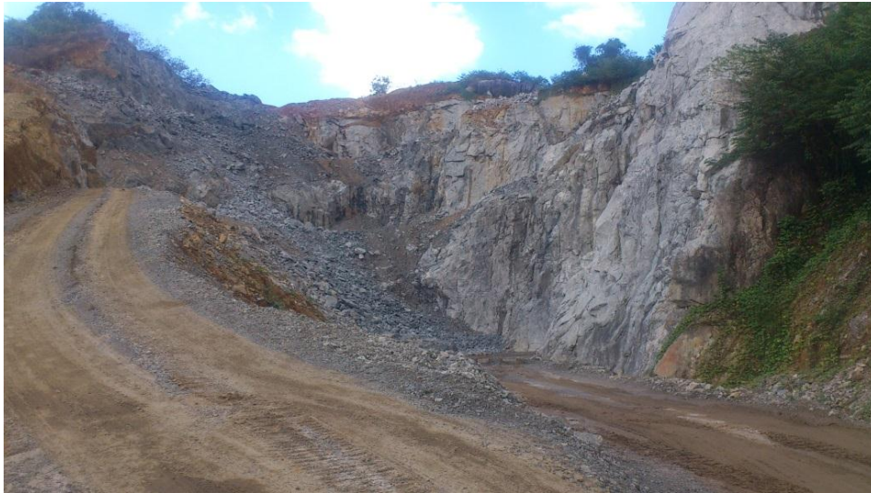
Figure 7.3: Part of the access ramp and working benches of the quarry no 03
