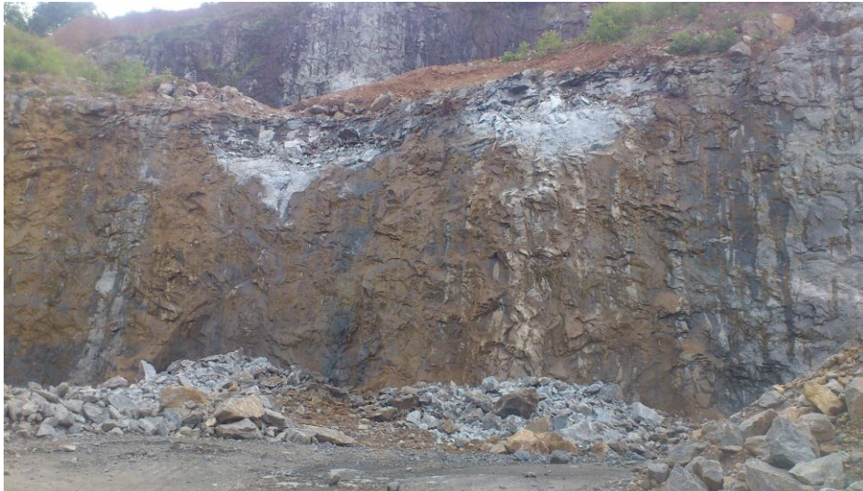
Figure 7.5: View of current blasting face of quarry no 05
