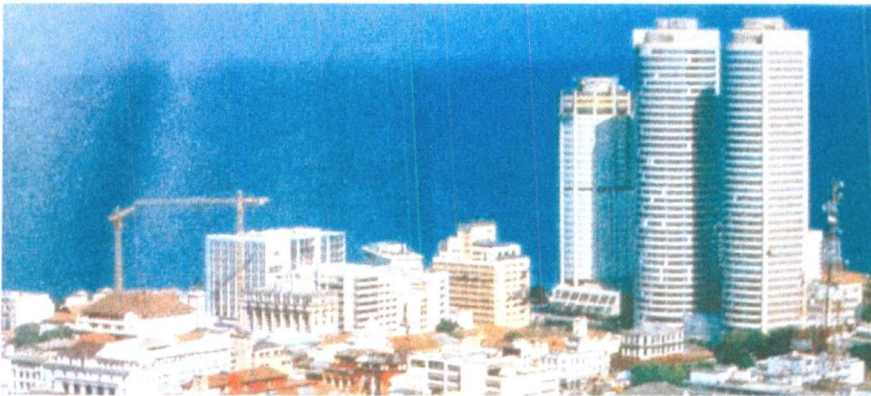
Plate: 1. 4 present developed condition in local city
