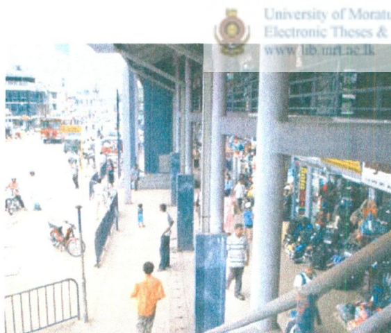
Plate: 1. 14 Building edge of the bus terminal Ambalangoda with Galle road
