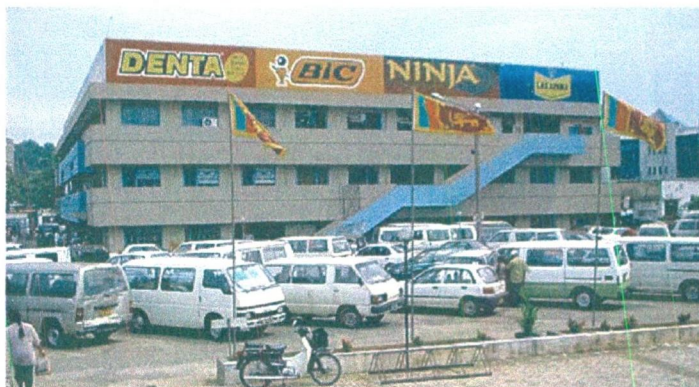
Plate: 3. 28 view from the open air theatre
