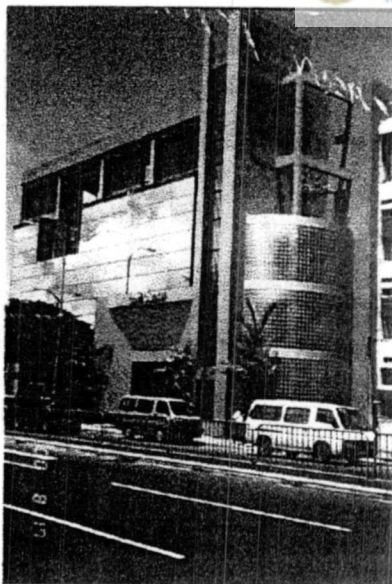
Plate 1.12b: the 'Avaranaya' building Colombo after renovation.
