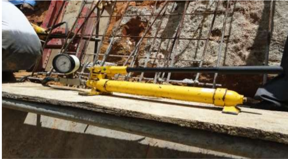
Figure 3.16 Application of pressure to the soil nail through the apparatus
