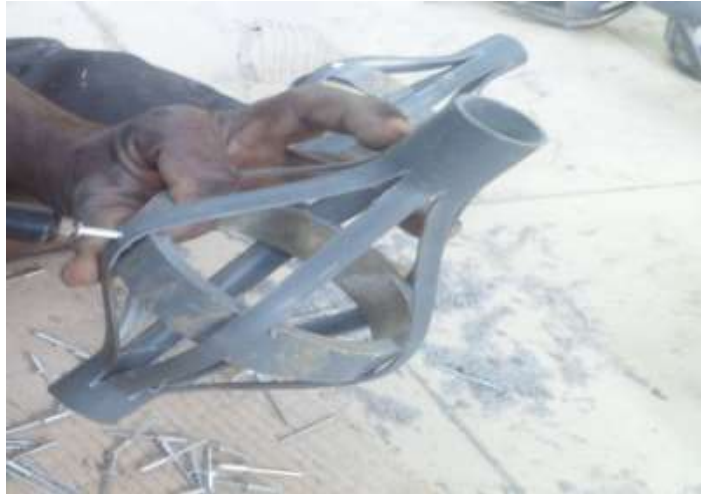
Figure 3.8 Preparing the 50mm cover with the use of 4” dia. centralizer
