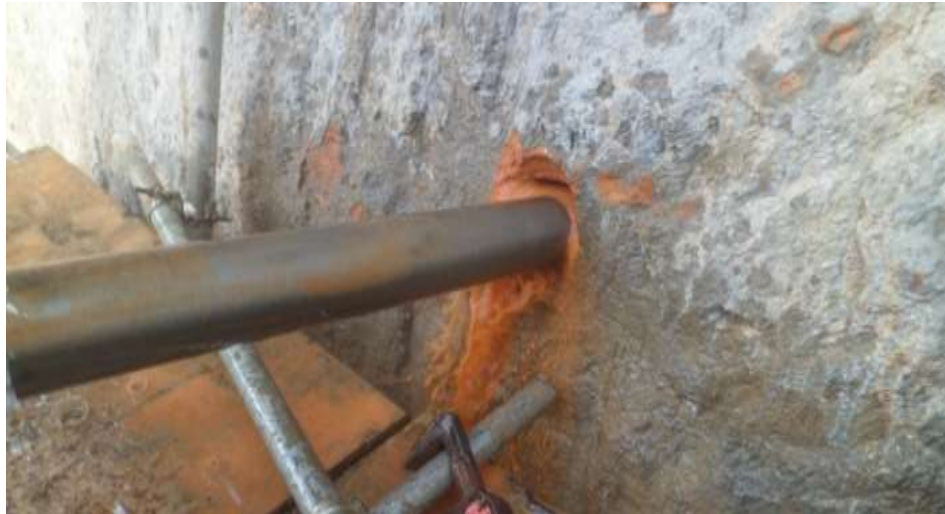
Figure 3.6 Shaft of the drilling machine
