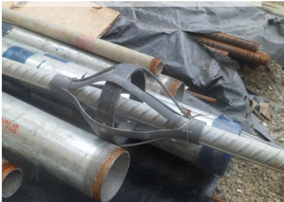
Figure 3.7 Galvanized soil nail with the PVC
