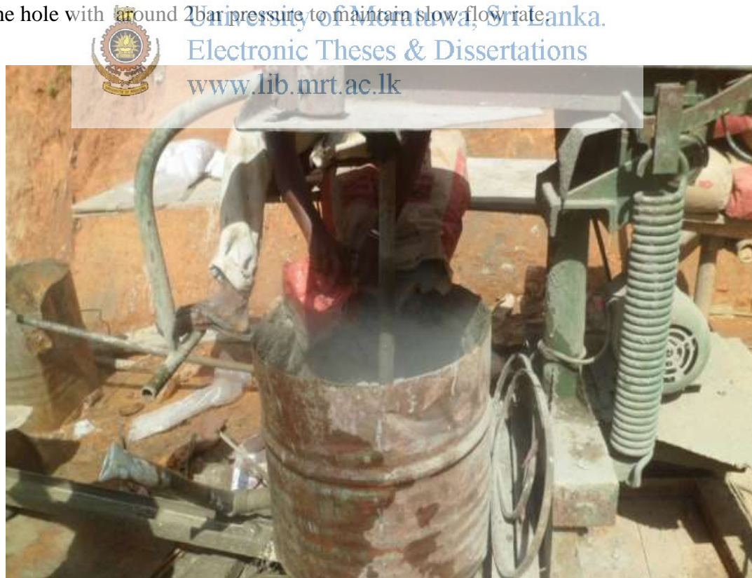
Figure 3.9 Cement and anti shrinkage grout being mixed in a barrel
