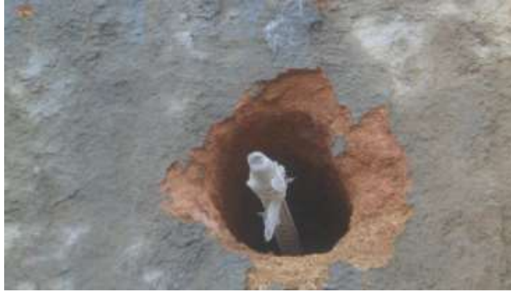
Figure 3.12 Grouted nail
