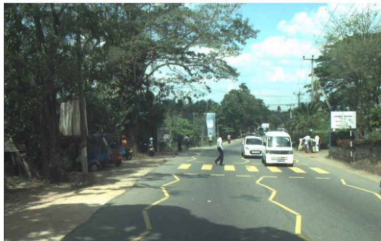
Figure 4.4 : Site Condition at Chainage 41+800 km
