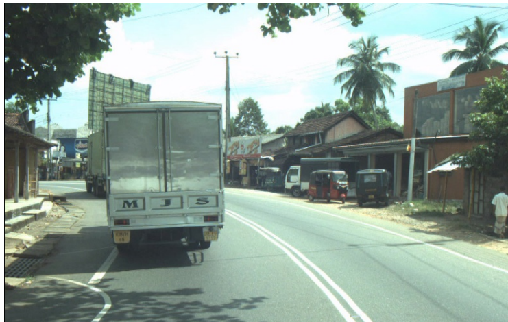
Figure 4.8 : Site Condition at Chainage 48+100 km
