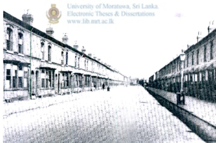
Figure 2.9: Whitehall Road – Birmingham (England)
