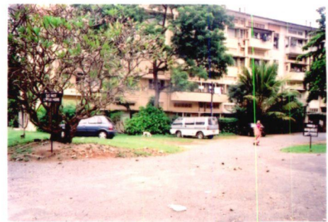
Figure: 3.5 the long blocks of flats to a height human scale with city living.
