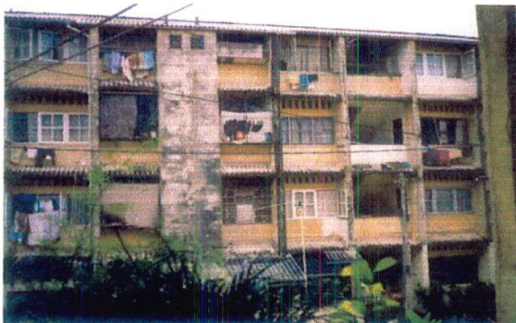
Fig 55: People add extra spaces to their house using the free spaces which was their as structural element
