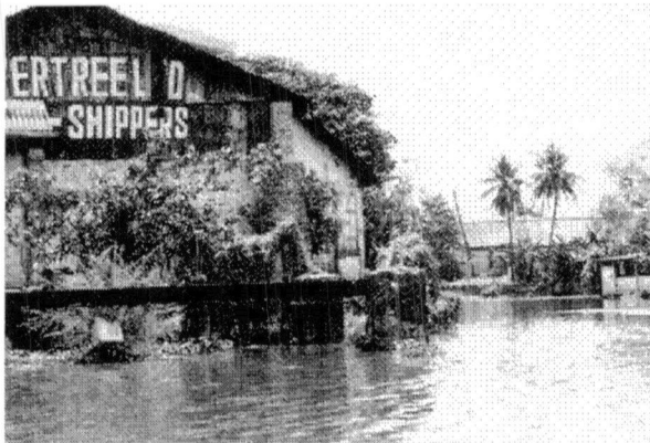
Fig. 84 East Beira Lake Entrance to inlet – area to redevelop
