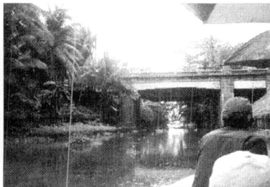
Fig. 142 Bridge at Galle Rd.
