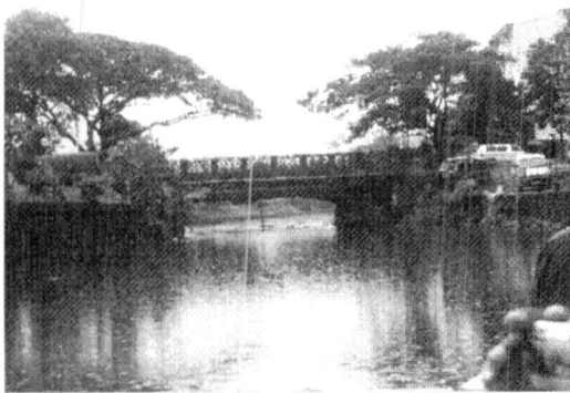
Fig. 140 Bridge at Havelock Rd
