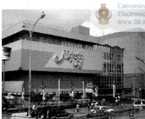
Fig. 23 Built fabric contributing to the street fabric
