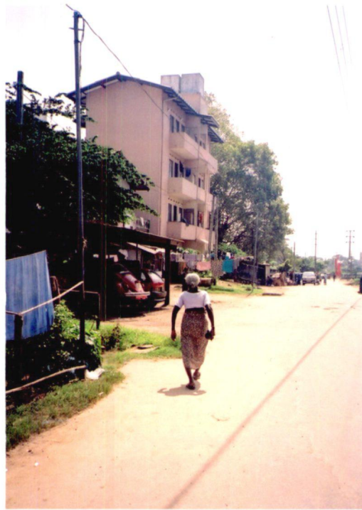
Fig 39. Home based socio Economic activities Garage interconnected to the house
