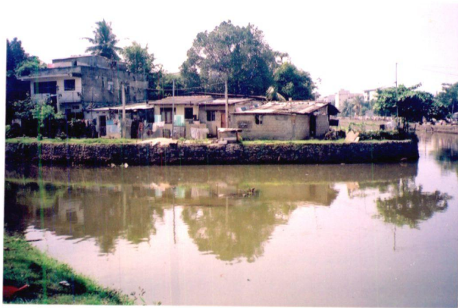
Fig 55. View of the Siddarthapura Housing settlement
