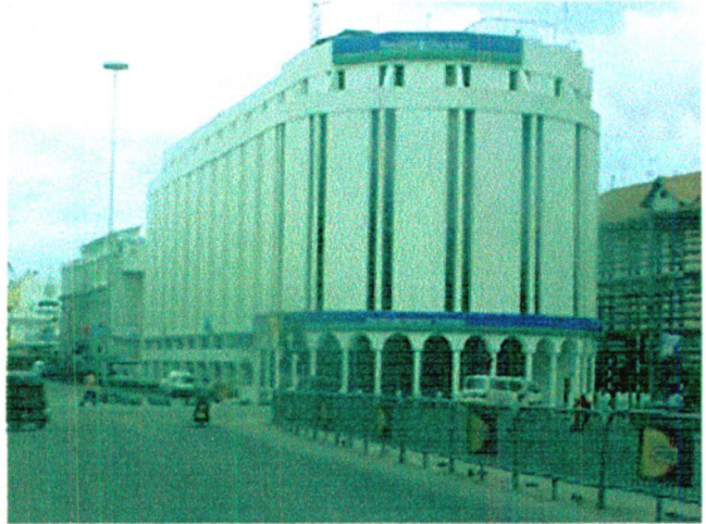
Figure 56 - Grinlays bank - expressive quality & the usage of materials of modernity.
