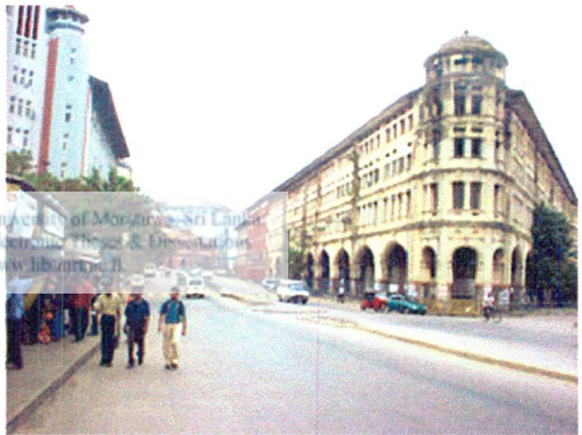
Figure 60 - Gaffur building responding to both roads.
