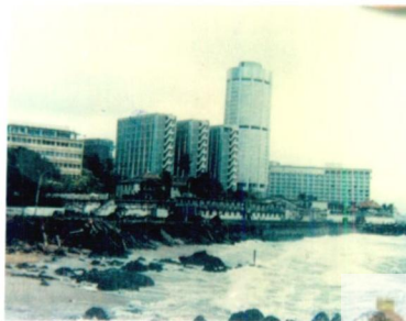
Fig.72 The abandoned buildings along the landside boundary.
