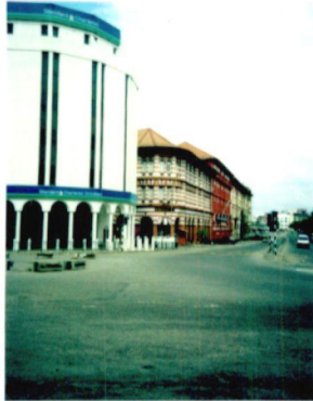
Fig.58 Facades rhythm totally fail in the Greendlays Bank.
