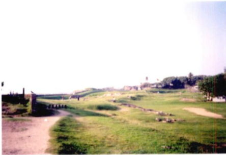
Figure 16. Large Open Area – Inside the Fort Used to place the Artillery Guns
