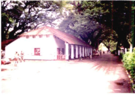
Figure 41. Tree Covered Road Inside the Fort
