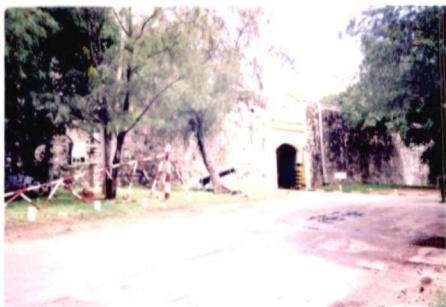
Figure 24. Entrance of the Fort Federic
