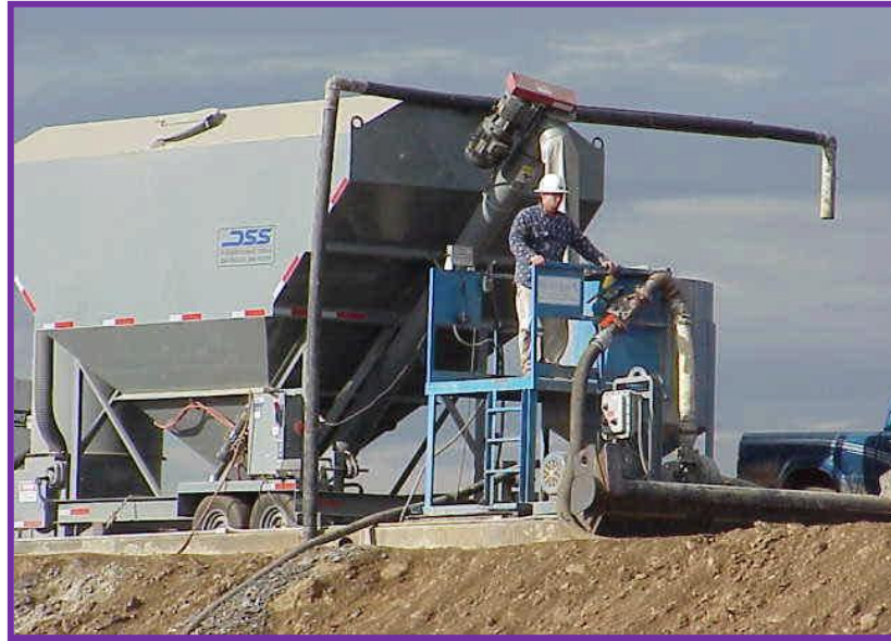
Figure 2.9 – Cement slurry preparing grout plant
