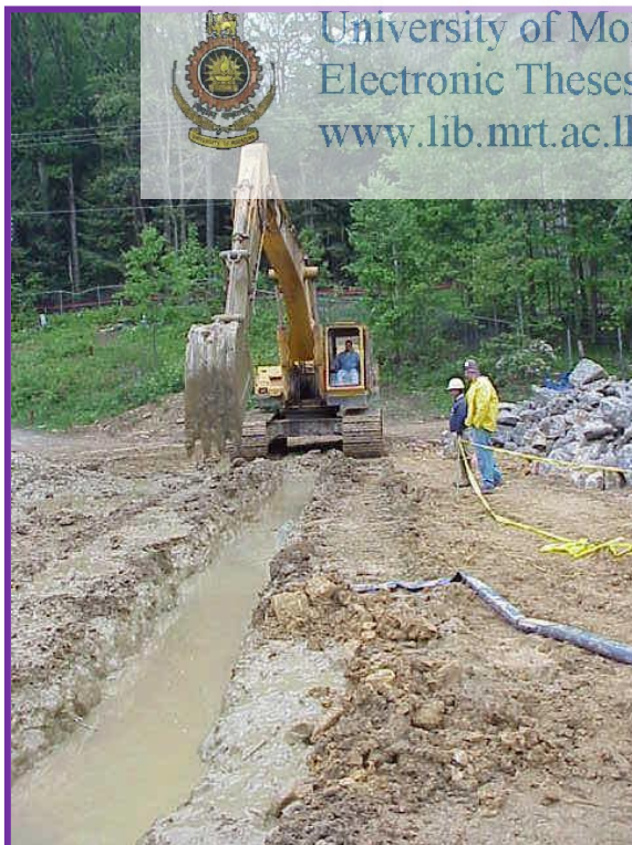
Figure 2.6 – Construction of Slurry Wall
