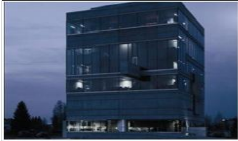
Figure 2.3: A well-controlled office building with lights turned off at night [7]
