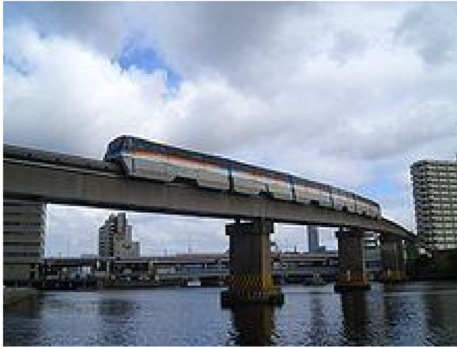
Figure 2.7: Tokyo Monorail system (Takahashi, 2014, http://www.akahabarnews.com ), (Original in Colour)
