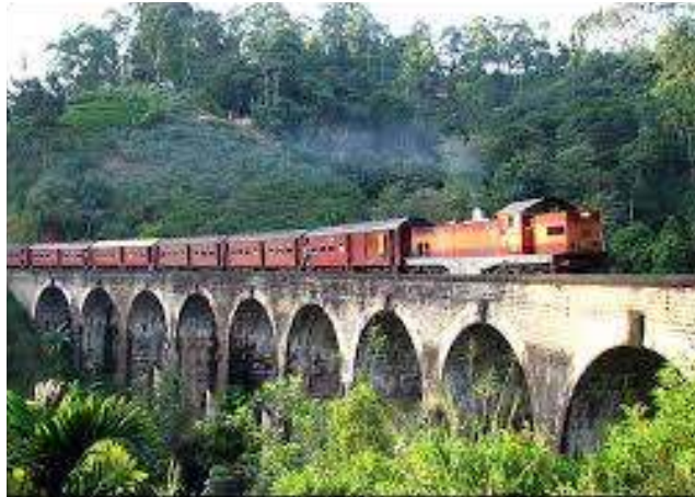
Figure 2-6“Nine arches” bridge on Badulla railway line
