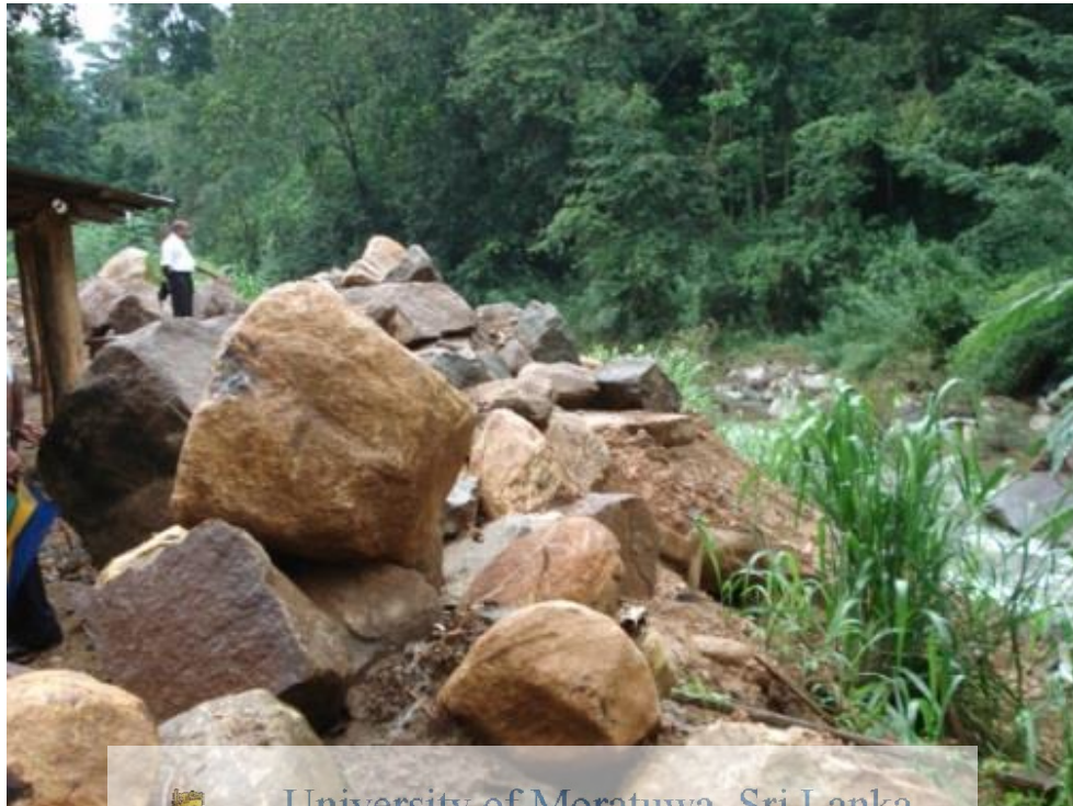
Figure 5.6 Spoil Rocks heap in the river bank
