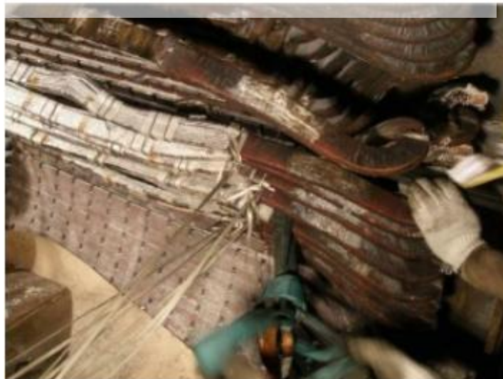
Figure 2.1 : Removing the damaged windings of GVPI stator at Tenau diesel plant
