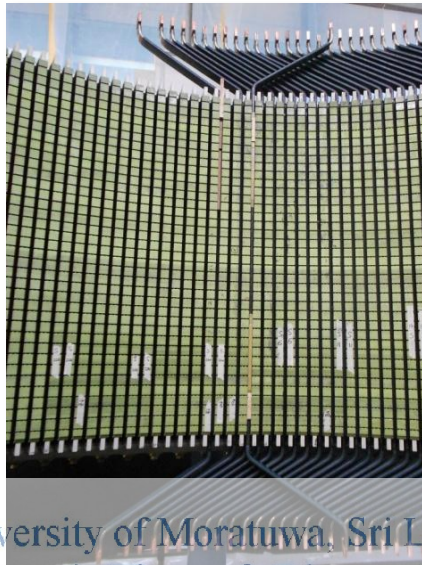
Figure 1.2 : Roebel bar windings of New Laxapana stator 'original in color'
