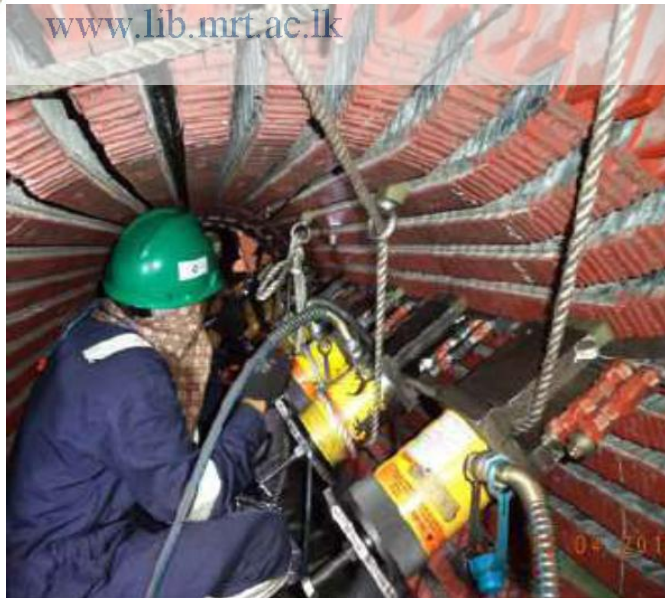
Figure 2.2 : Removal of the winding bars using hydraulic jacks
