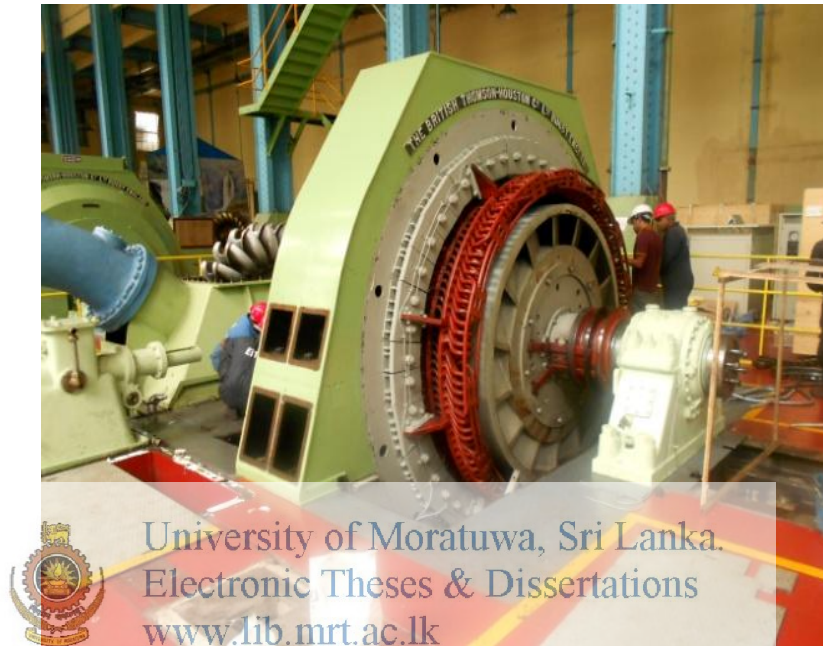
Figure 3.4 : VPI stator of Old Laxapana 'original in color'
