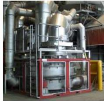
Figure 3.3: (a) Rotary Regenerator, (b) Rotary Regenerator on a Melting Furnace [16]
