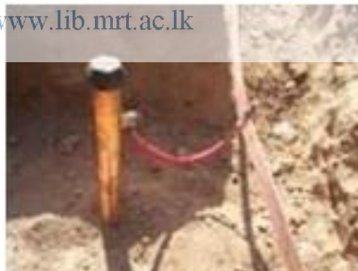
Figure 6.2: Chemical rod installation in space restricted places
