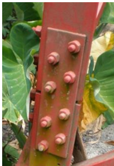
Figure 3.4: Tower leg joint
