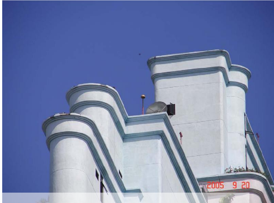
Figure 1.11: A view of the Villaputti building from a different angle. Since the curved edges had been struck by lightning repeatedly, the claimed existence of the collection volume is doubtful.
