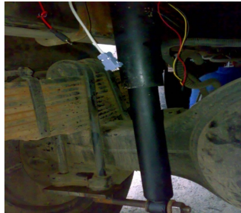
Figure G6: Wiring the system
