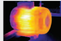
Motor: Internal Winding Problem
