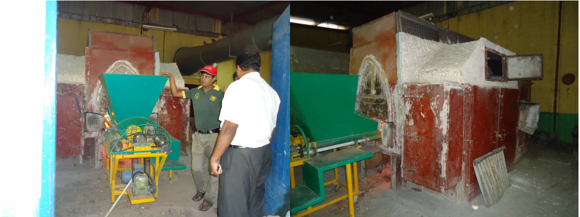
Figure 7.2: Hot air generator after retrofitting
