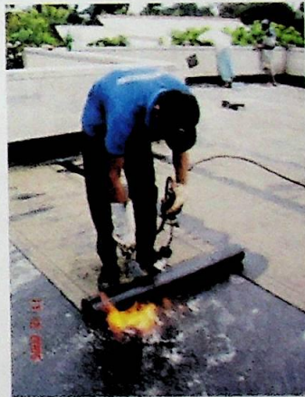
Figure 2.7: Application of Torch on membrane
