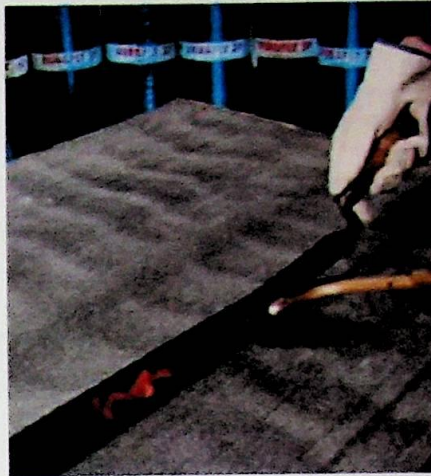
Figure 2.8: Preparation of Joints ( www.nuralite.com )
